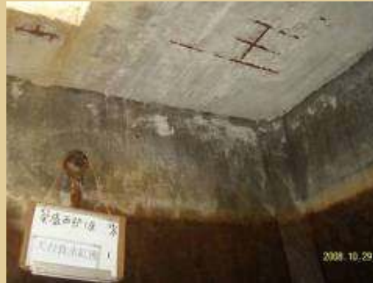
EXISTING FAIR-FACE FINISH INSIDE THE WATER TANK
