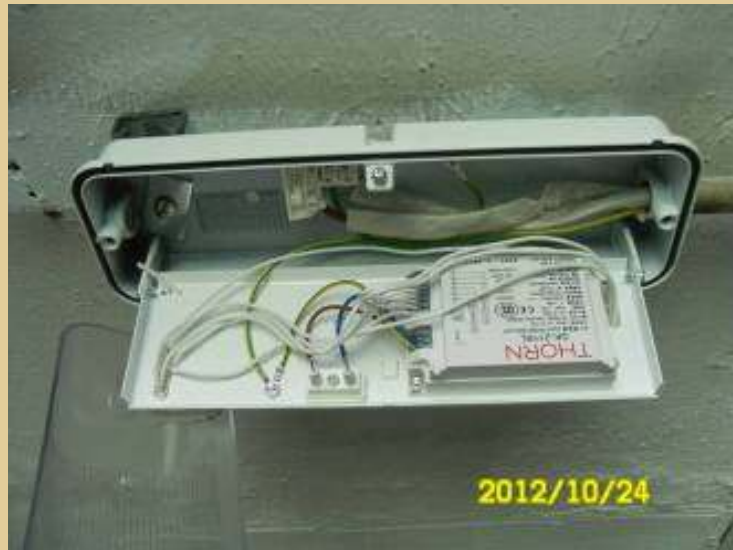
BULKHEAD LIGHT FITTINGS C/W ELECTRONIC BALLAST
