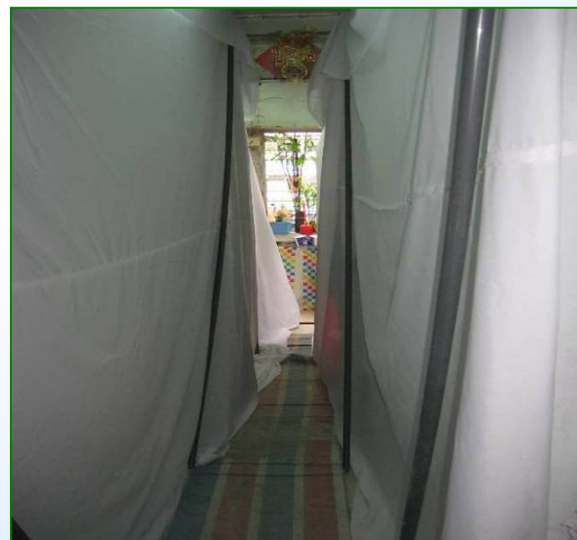
Dust Screen Protection inside Tenant's Flat
