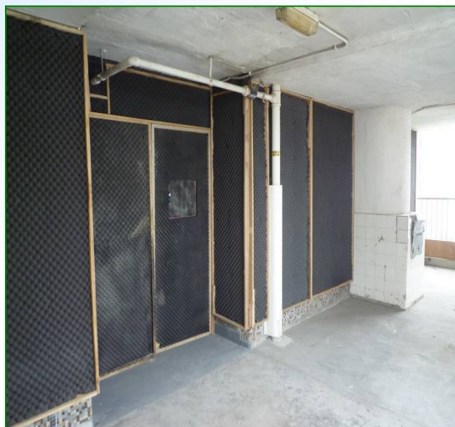
Noise Absorbing Panels enclosing Works Areas
