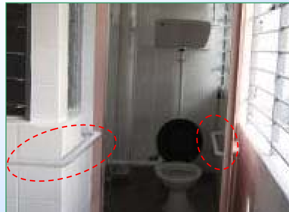
Handrailing for Elderly and Disabled
